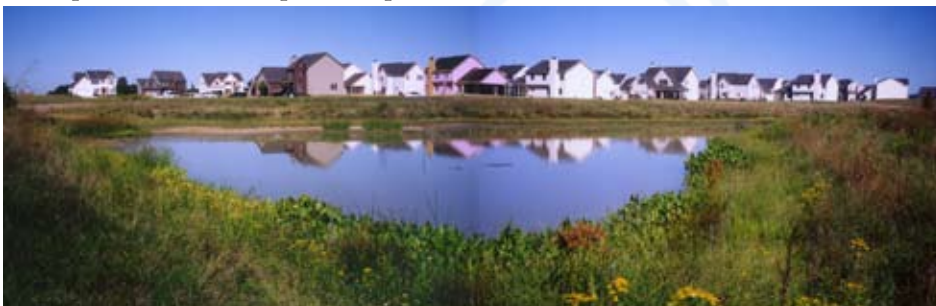
Bioengineering materials and native plants were installed by JFNew along the edges of this retention pond for a residential subdivision in central Indiana.
